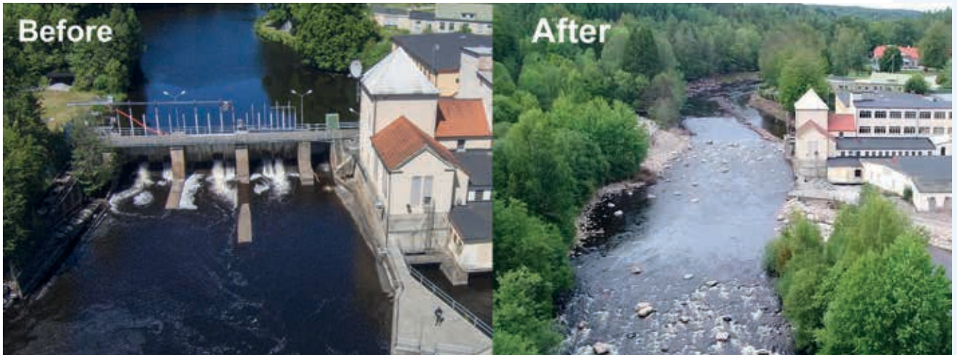
An example of river restoration within the LIFE CONNECTS project showing the removal of Marieberg hydropower plant in Mörrumsån. © Uniper
