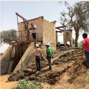
Installation of the station in Kollo
