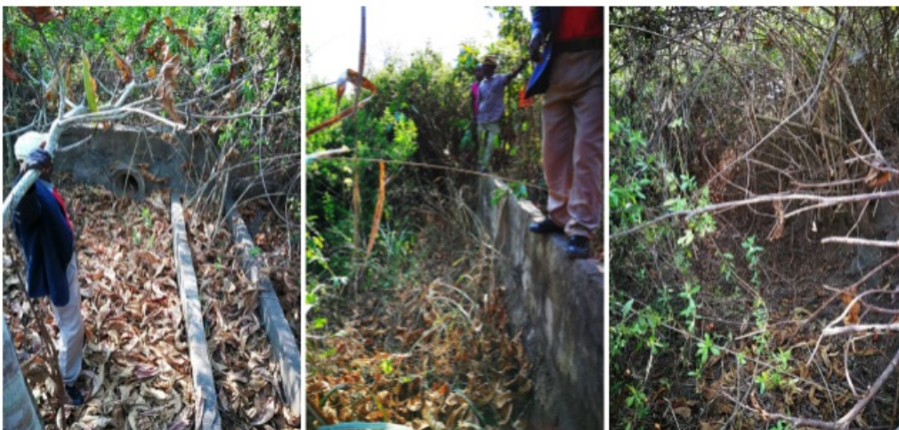
Some examples of the current state of irrigation infrastructures and rehabilitation
