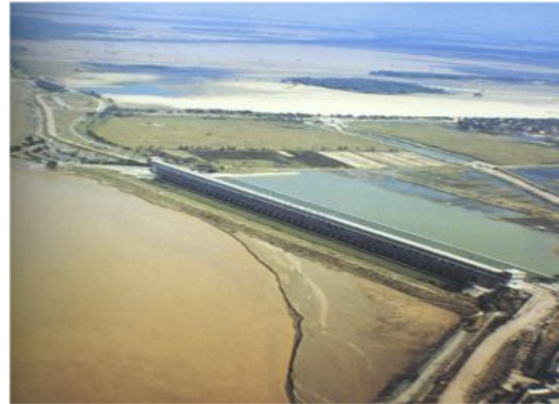
Dongping Lake flood detention basin
