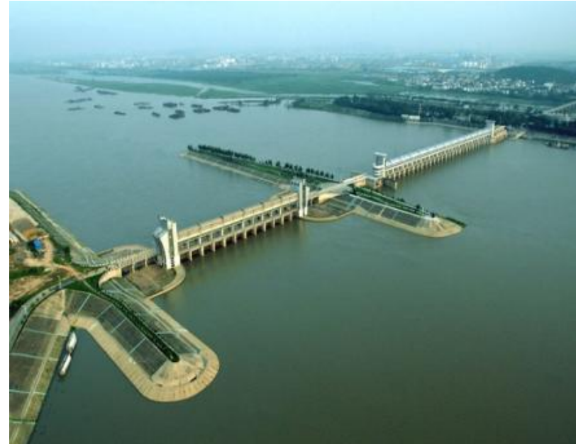
Bengbu sluice on Huai river
