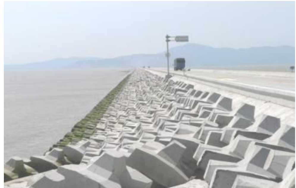
Sea embankment in Zhejiang province
