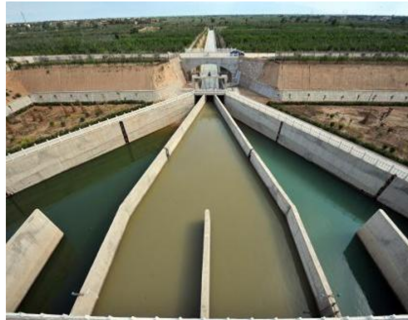
Canal of Jiamakou irrigation district in Shanxi
