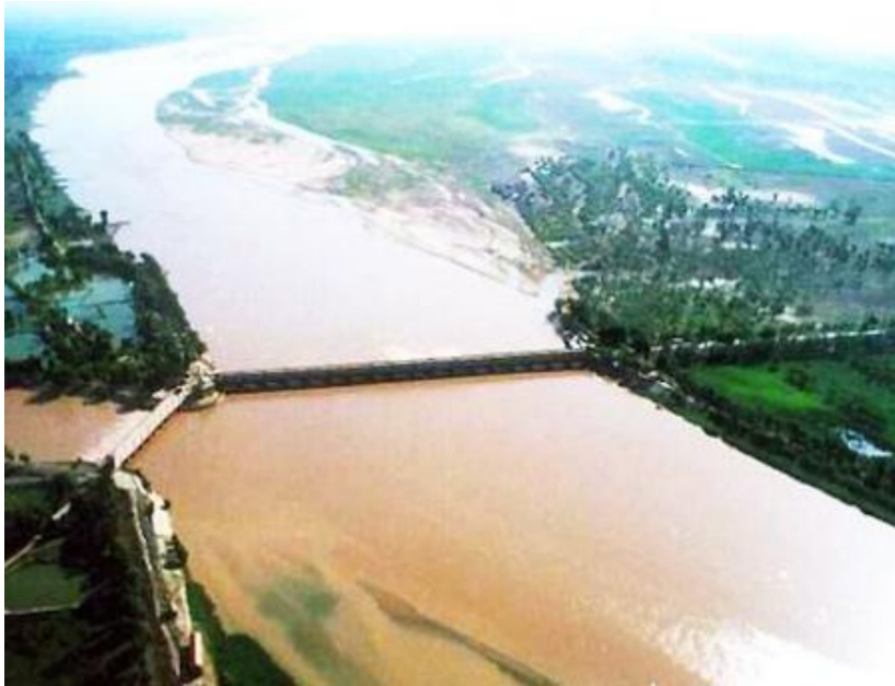
Sanshengong sluice on Yellow river
