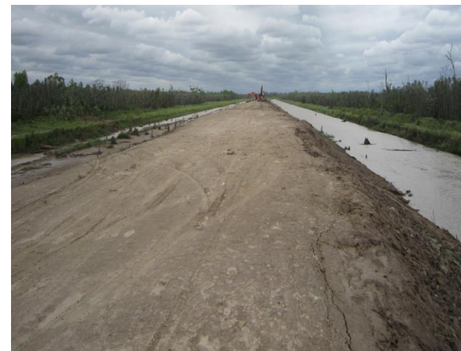
STRUCTURAL MEASURES: longitudinal embankment
